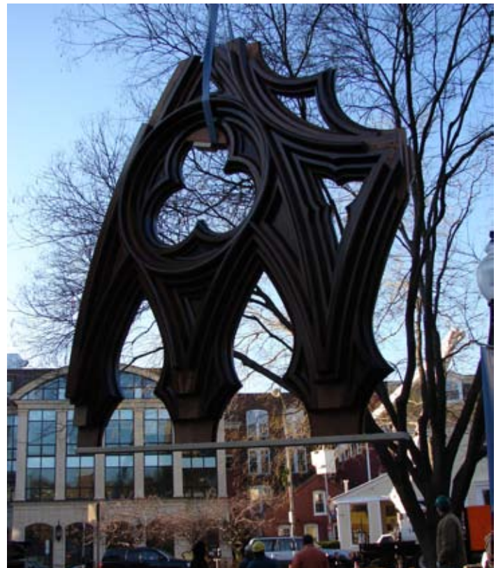
"A view of the installation process shows just how large a project can be created on a Cabinet-Shop router." ►
