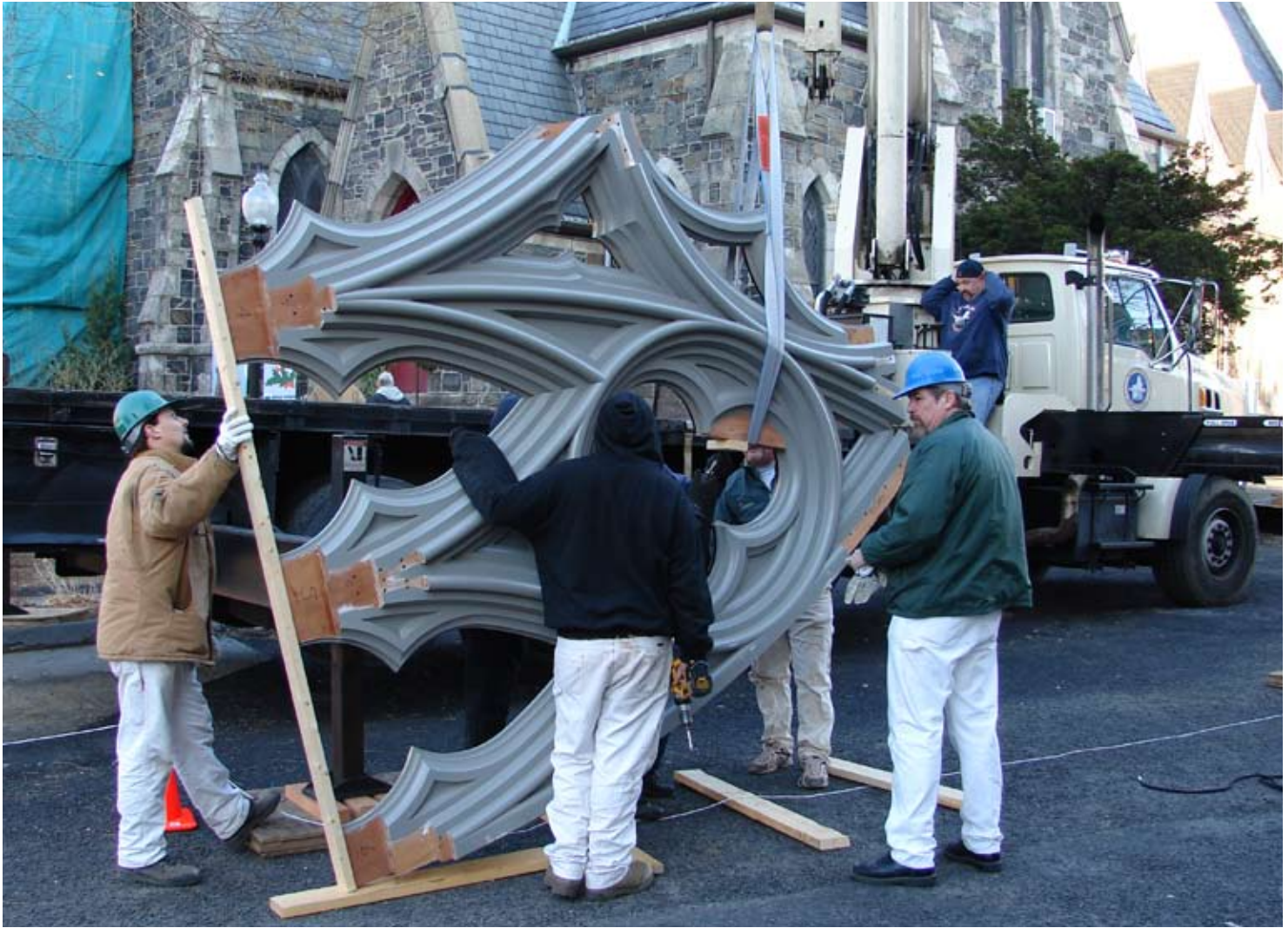
"Kingsland Corp uses a Thermwood CNC router to create some truly stunning projects like this elaborate church window." ▲
