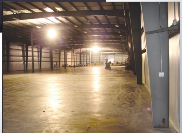
Interior of our new production area waiting for lights ▼
