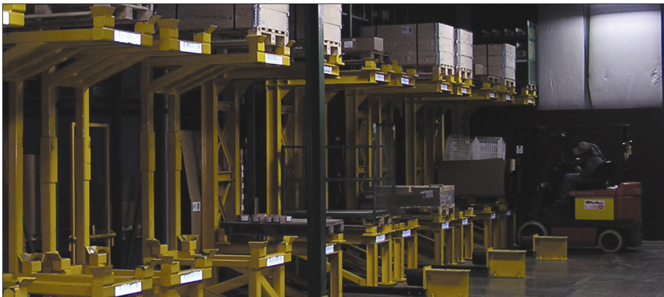
Häfele's automated high rise storage has the same capacity as a quarter million square foot warehouse but is far more efficient
