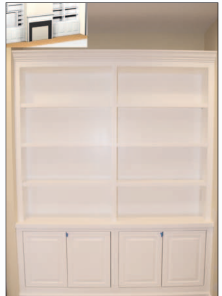
Wayne's wall design (upper left) and one side during construction ►
