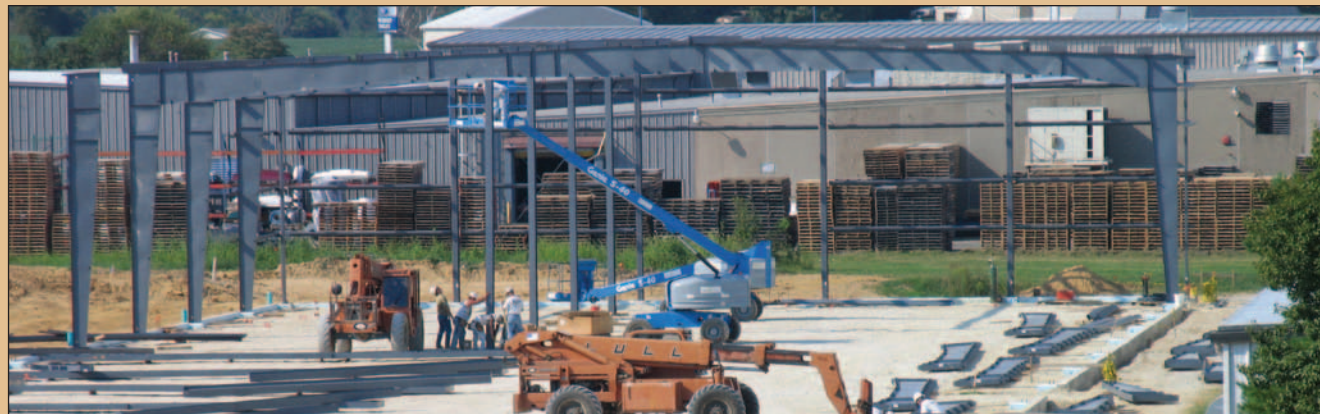
Starting to erect the steel
